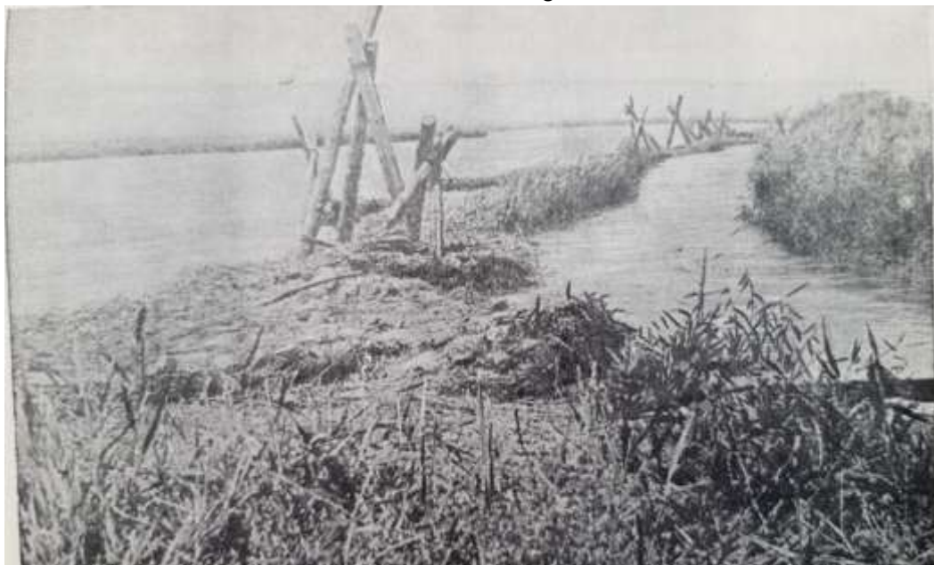
Figure 1. Water from the river is directed into the canal using flow-deflecting barriers of the “Sepoya” type.
