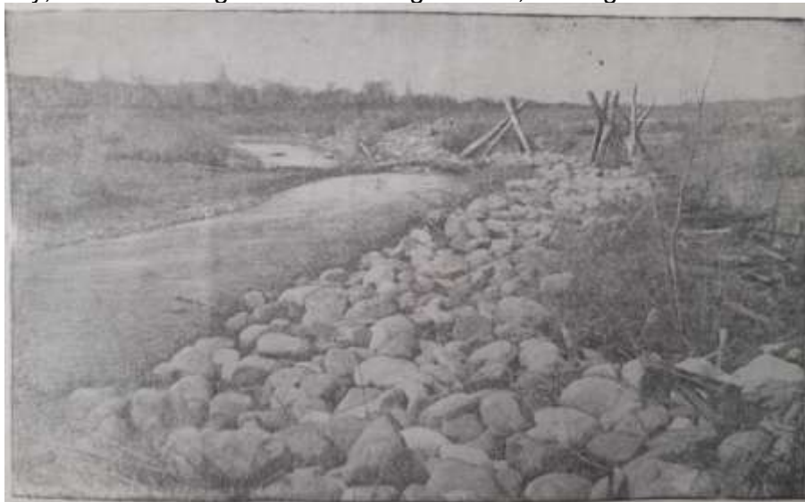
Figure 4. Stone and shrub (rock-dam) embankments built to protect canal banks from erosion are reinforced with sepoyas .
